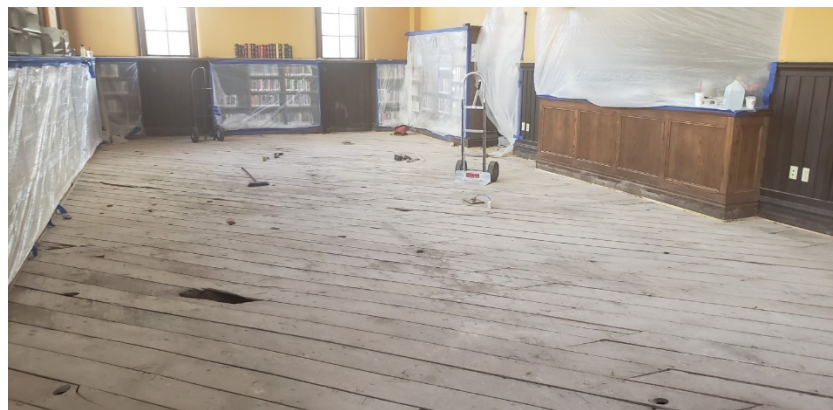
Old Colorado City Flooring - North demolition
